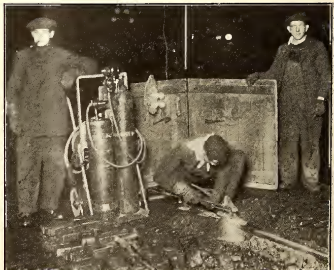
TRACK REPAIR GANG WORKING AT NIGHT
